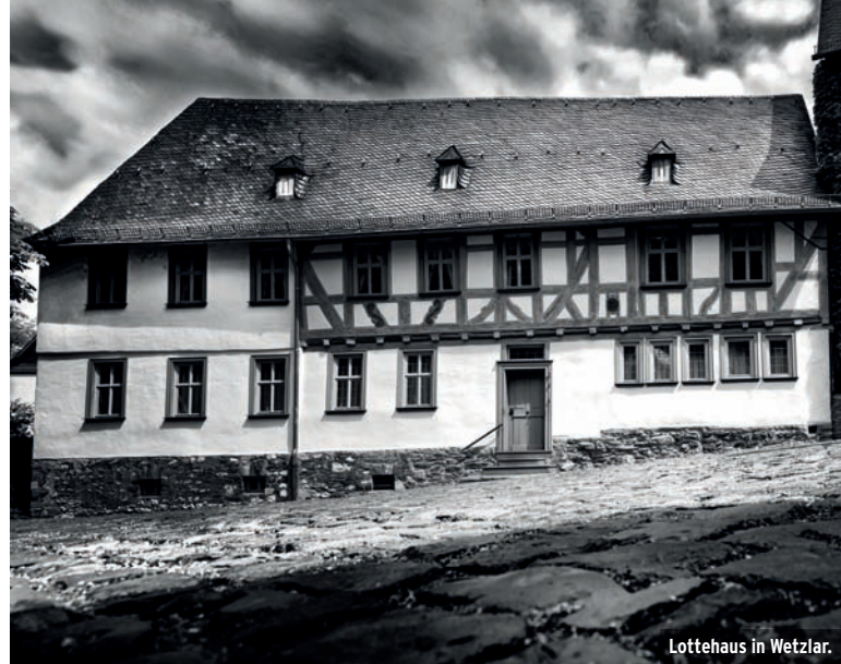
Lottehaus in Wetzlar.
